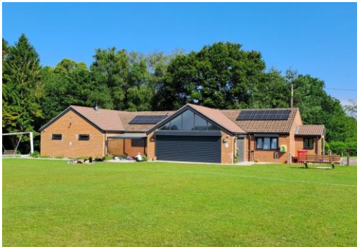
Shedfield Recreation Ground Pavilion extension
